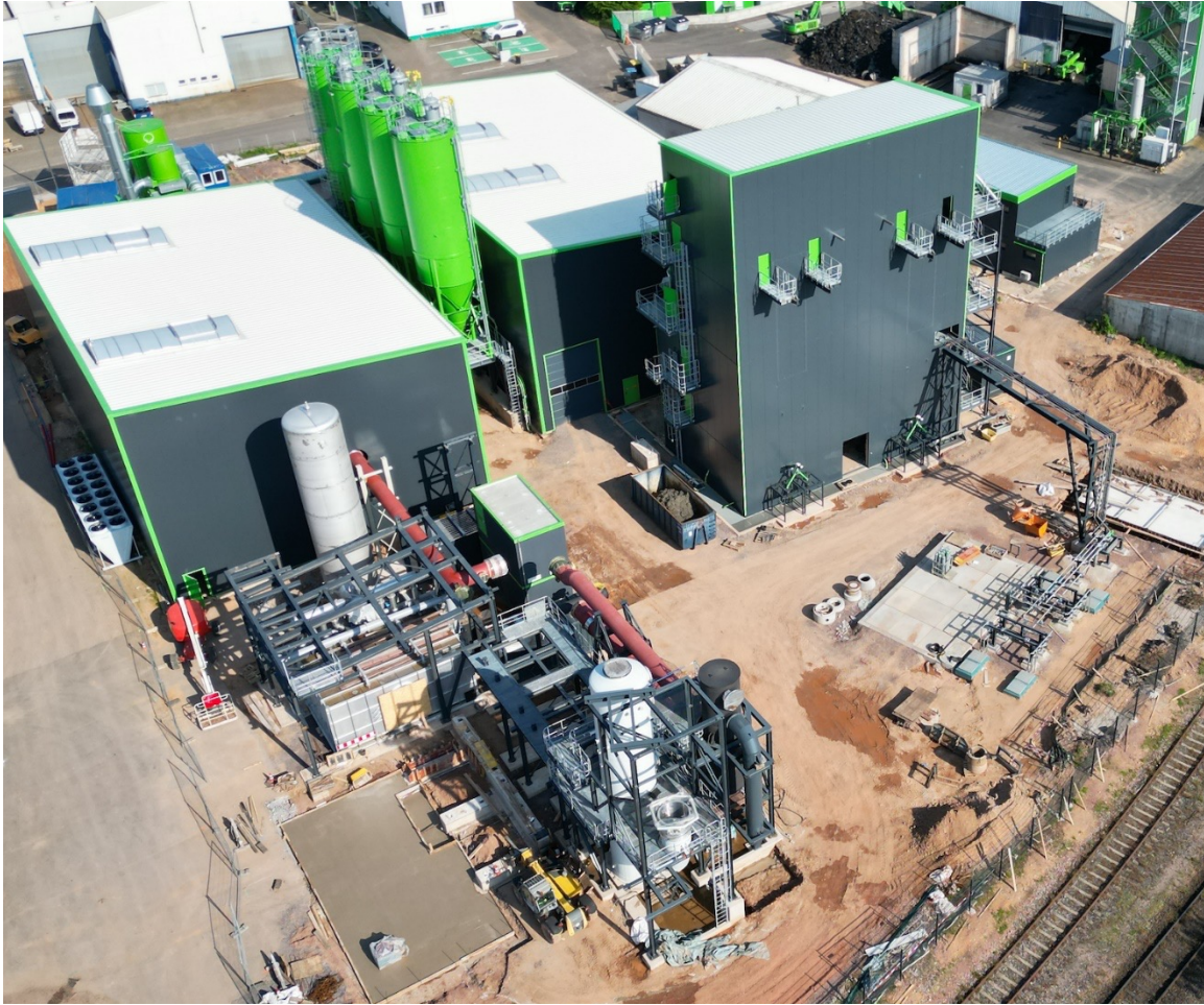
Back view with Power Plant / Oil Storage and Pyrum Tower
